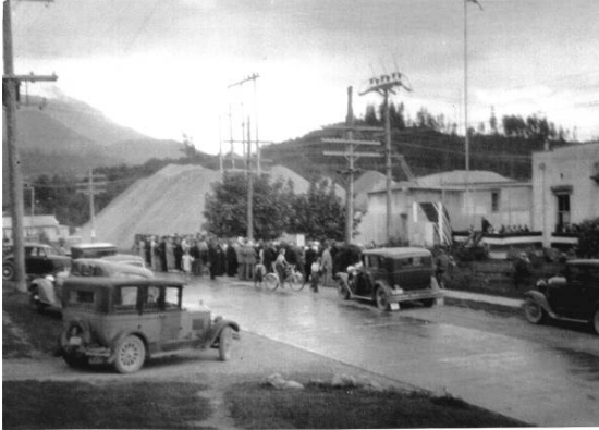
Dedication of the Superior Office Building – photo from S. Hager
